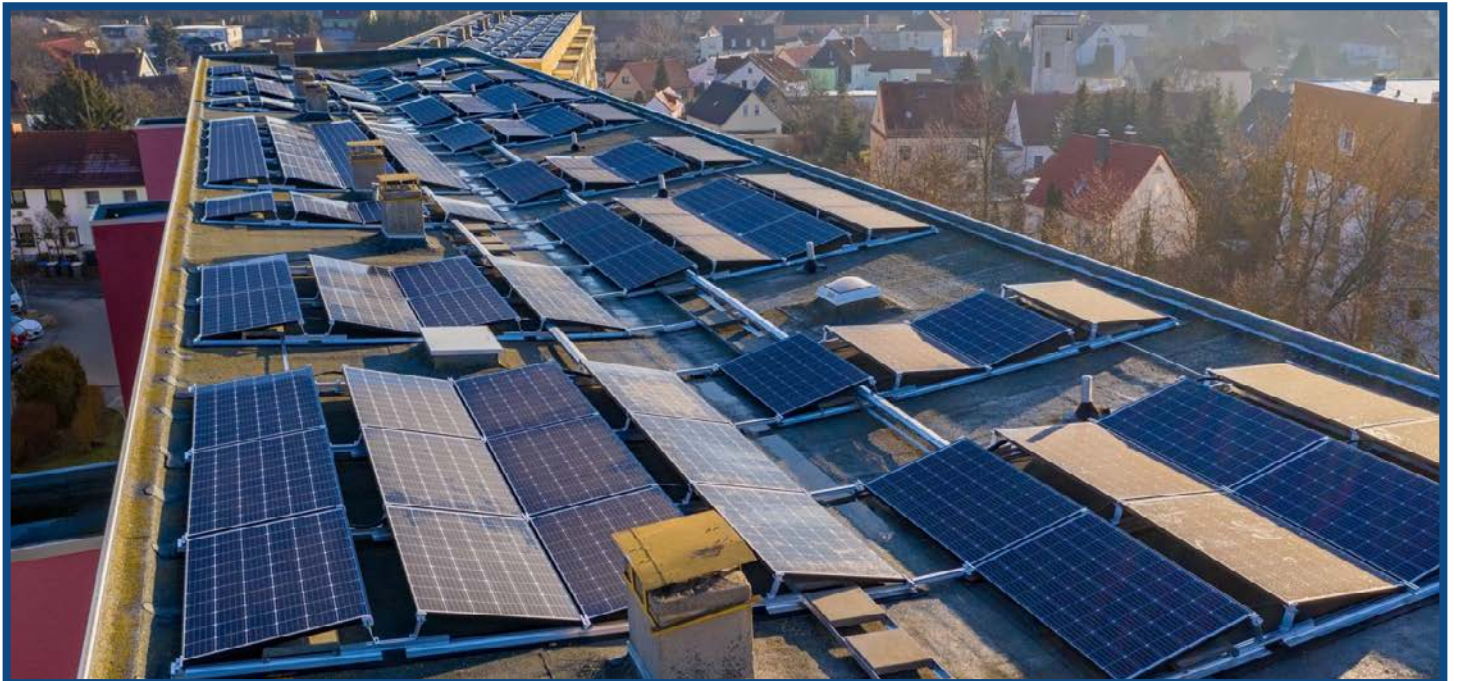
Credit: YSG Solar ballasted rooftop system
